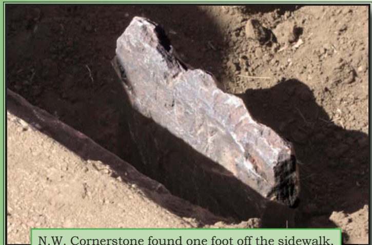
N.W. Cornerstone found one foot off the sidewalk, clearly marked with chiseled "NW"
